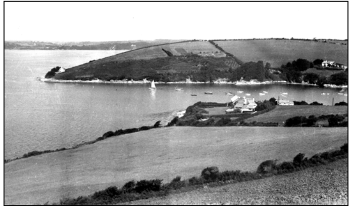
The Creek in the early 1950s. Only Bar Point, Trecarrell and Point House can be seen on this side of the Creek. Messack House has no staff quarters and you can clearly see the cottage on Messack Point that was demolished in c. 1970.
